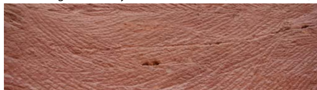
Tool marks from iron picks on the quarry face.
