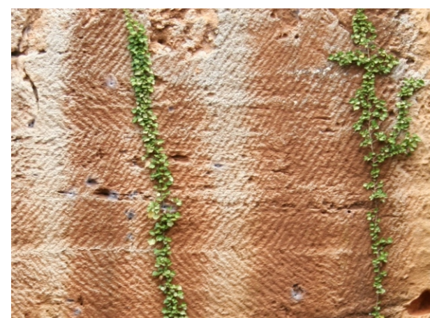
Tool marks from quarry picks on the vertical quarry faces
