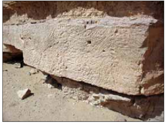
b: Quarry marks showing the probable use of picks within St. Simeon's monastery
