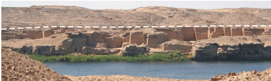
Open cast sandstone quarries situated in a horizontal layer of good quality sandstone (upper limit marked with the dotted line). Gebel el Silsila, Egypt.
